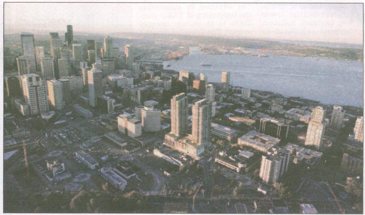
Nearby office buildings could export heat to residential buildings like the Insignia (center) if the city had the right infrastructure. The two-tower complex will have more than 1,000 heat pumps, but will still need natural gas to assist with heating. Image courtesy of Embassy Development
